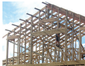
A Building under Construction
